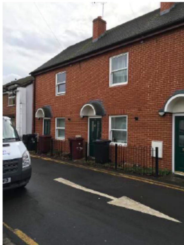
Modern terrace development at no.s 2, 4 and 6 Eldon Terrace
