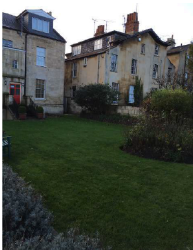
Rear of numbers 15 and 17 Eldon Square Front elevation of 17 Eldon Square
